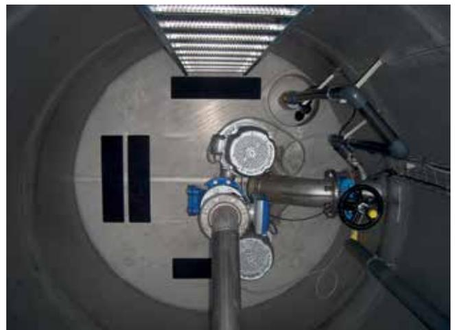
Sidinix prefabricated lift station fitted with the DIP System
